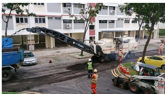
*The road surface is removed and a new bitumen layer is added*
